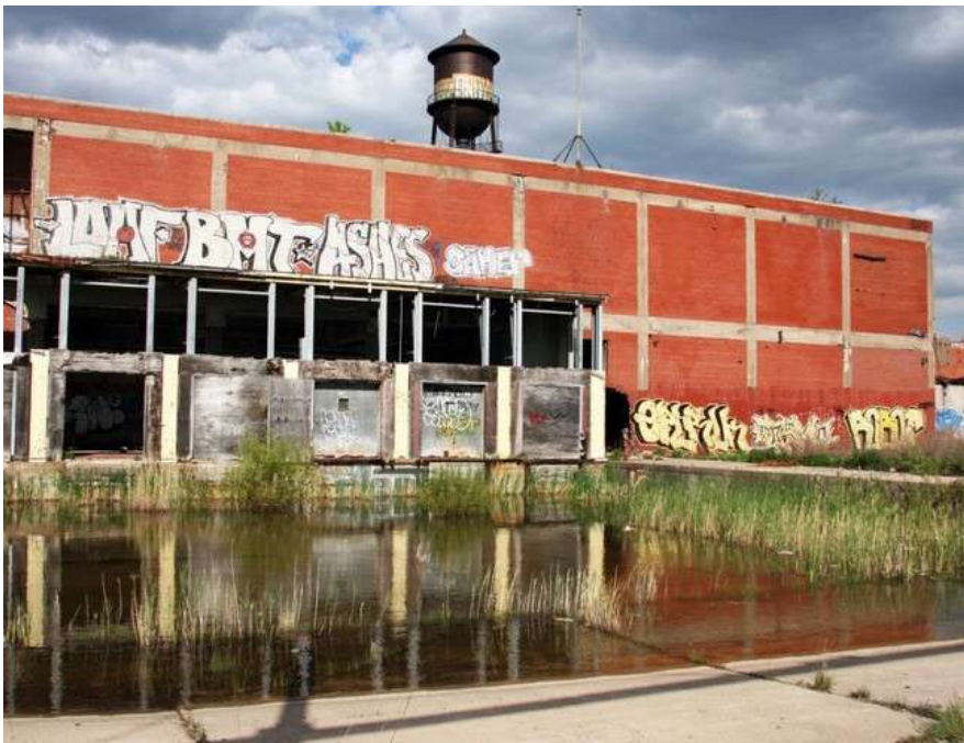
Fig. 11 A functional wetland dominated by reed developed in an unoccupied factory.
