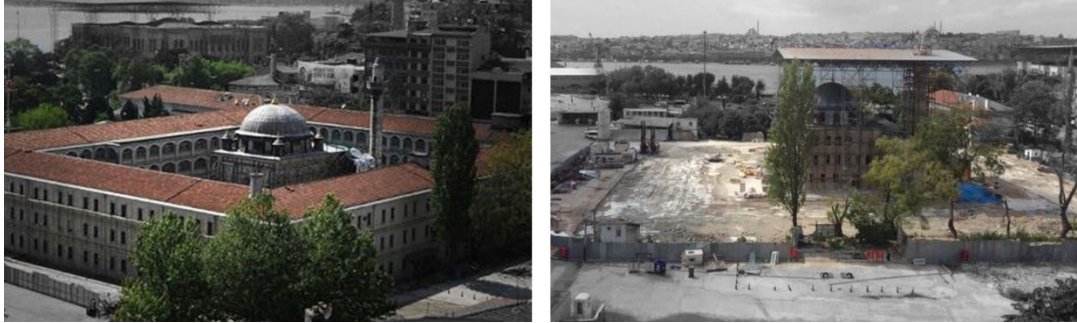
Fig. 31 Kalyoncu Barracks before and after demolition.
